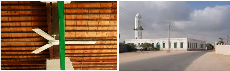
Figure 3. This is the Turkish Mosque. The ceiling is made of wood, while most buildings in Berbera use steel ceilings, which makes the mosque cooler during the summer.
